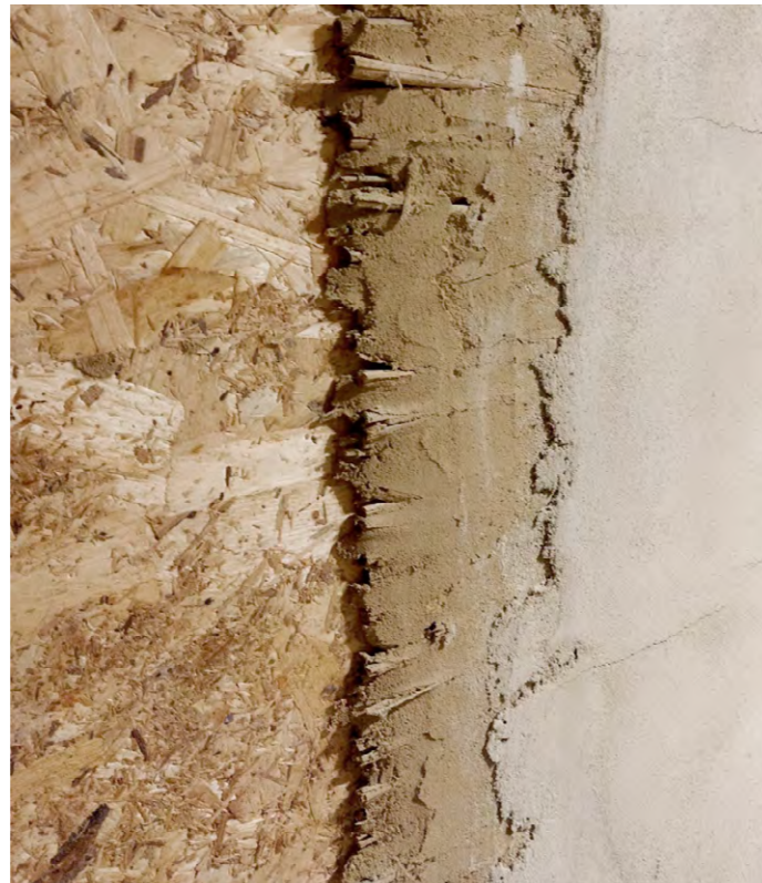
OSB panels with reed lath stapled on it. The reed lath should be covered sufficiently (more than on this image) to create a homogenous base coat and avoid cracks
