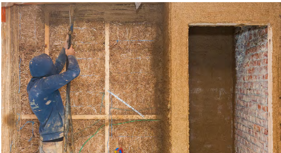
Léém Clay plaster applied with a spraying machine on reed lath, strawbale and masonry
