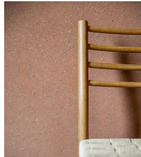
Natural sand present in the Léém Clay Plaster becomes visible as a result of excessive sponging
