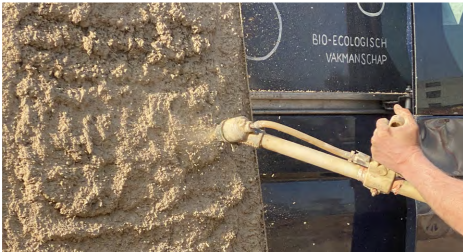
Léém Clay plaster applied with a spraying machine
