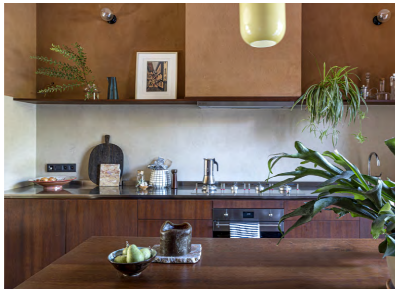
A Léém Clay Finish Red in a kitchen area (on top). At the splashback zone a cream Léém Finish with added waterproof casein layer (available in the Léém product range) has been applied.
