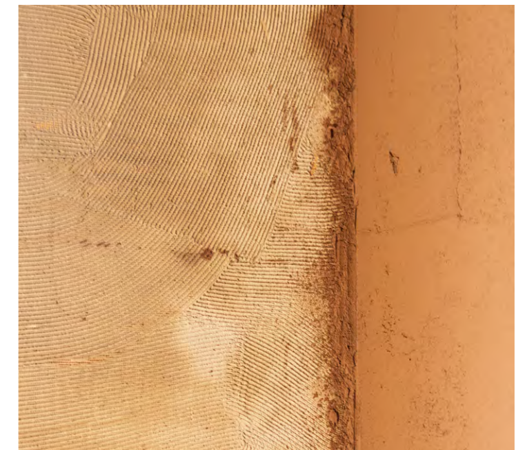
Léém Clay Plaster Brown as a basecoat in rough texture, Léém Clay Plaster Red as a toplayer
