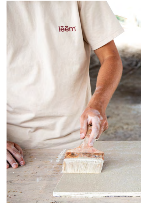
Application of the Léém Clay Paint with a wide brush
