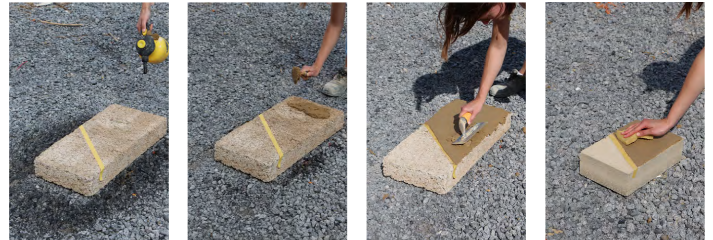
Different steps of plaster application
