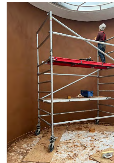
Scaffolding for manual application of Léém Clay Plaster
