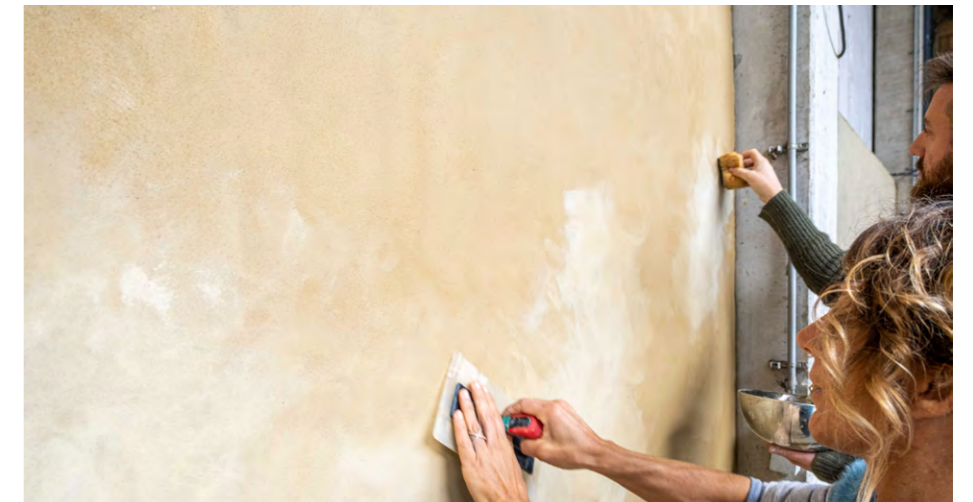
Using a plastic flexible trowel allows to reach a polished smooth surface
