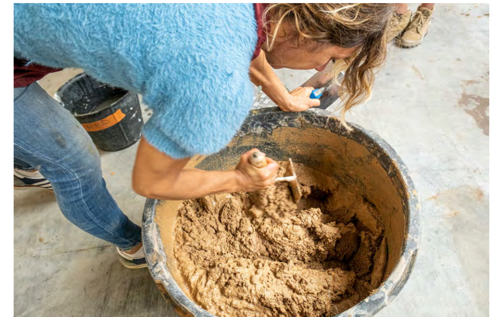
Preparation of Léém Clay Plaster
