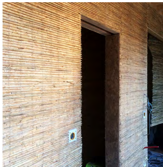
Reed lath stapled on OSB panels at project Karper, Brussels
