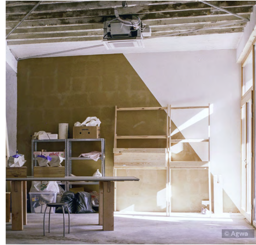
One base coat of Léém Clay Plaster Brown on top of hempcrete masonry. The ghost lines of the masonry joints shine through. To avoid this, at least two coats are needed.
