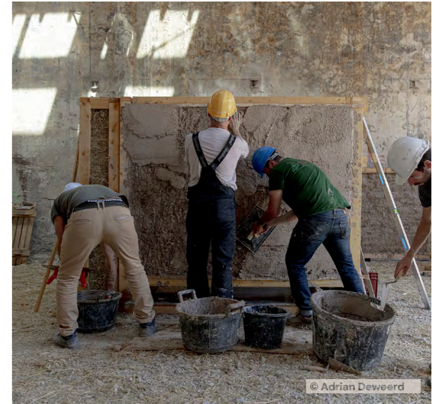
Prototype of clay plaster on straw bales
