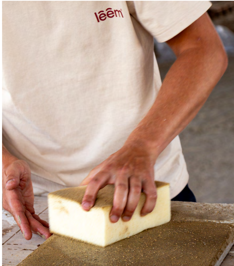
Clay plaster with a large amount of straw fibre
