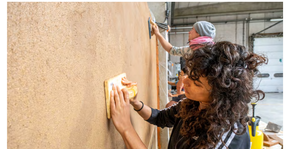
Using a wood float results in a well densified surface
