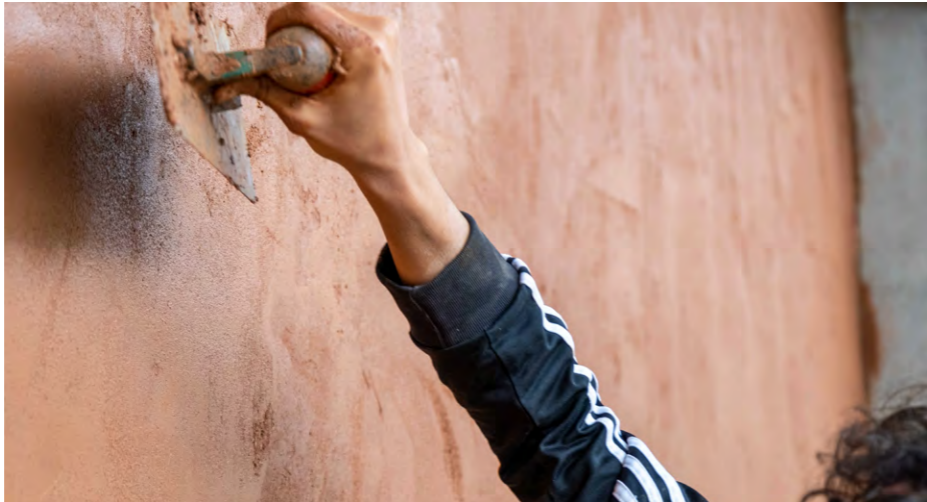
Léém Clay plaster applied manually with a trowel
