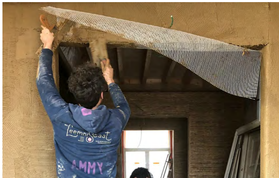
Léém Flax Reinforcement Mesh embedded in the base coat, covering the lintel
