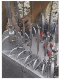
Detail: cable connectors at base of the central 'bouquets'. These cables are not load bearing, structural and vines are trained directly onto the cables.
