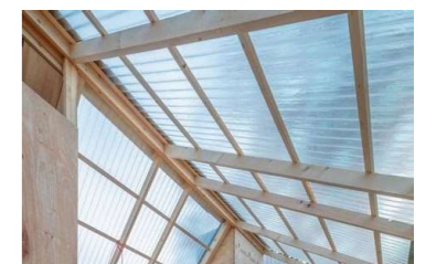
Roof: corrugated transparent sheet
